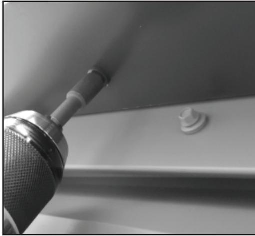
12. For 3' and 4' cupolas only with formed metal corner gussets: Using #10 x 1" self-drilling fasteners (provided), install 2 fasteners through underside of overhang of each roof side approx. 8" from each corner and 2" from the roof edge to pull the roof overhang and corner gusset together.
