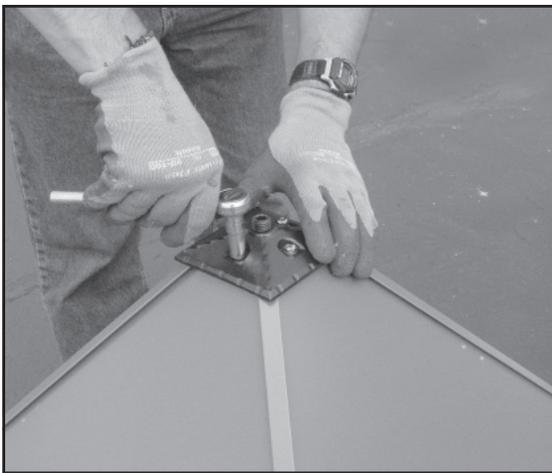
9. After all the roof connectors are pushed up under cap, tighten the bolts on the roof cap to complete the assembly. Caulk over each head to prevent possible leaks. Trim the roof connectors off at the bottom to create a finished appearance.
