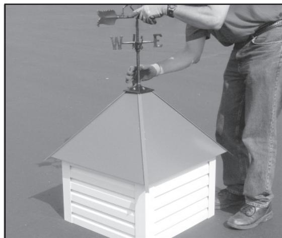
10. If a weather vane is being used, remove threaded insert and take care to properly thread the mast into the threaded hole in cap.
