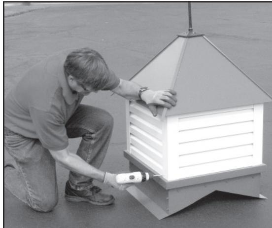
11. Attach the completed cupola to the base with fasteners to complete the installation. Predrill 1/8" holes for best appearance. (On 48" model be sure to screw through center blade stiffener).
